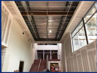
Ceiling grid and hard ceilings being installed in lower level monument entry
