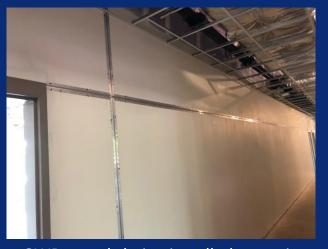
GWB reveals being installed on main west (corridor C1-2)
