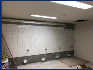
Ceramic tile install in lower level gang restroom
