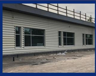
Metal panel installation on Elevation F-1 (3<sup>rd</sup> level)
