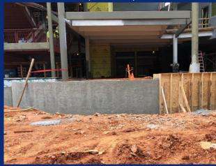
Radius retaining wall B formed and poured at terrace entrance
